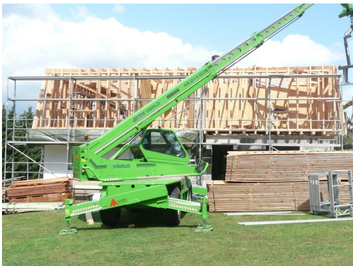
Monter la charpente
